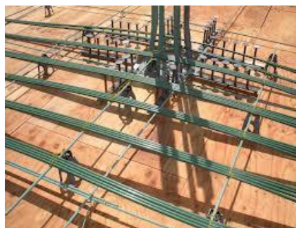
▪ Mono strand post tensioning reinforcement
